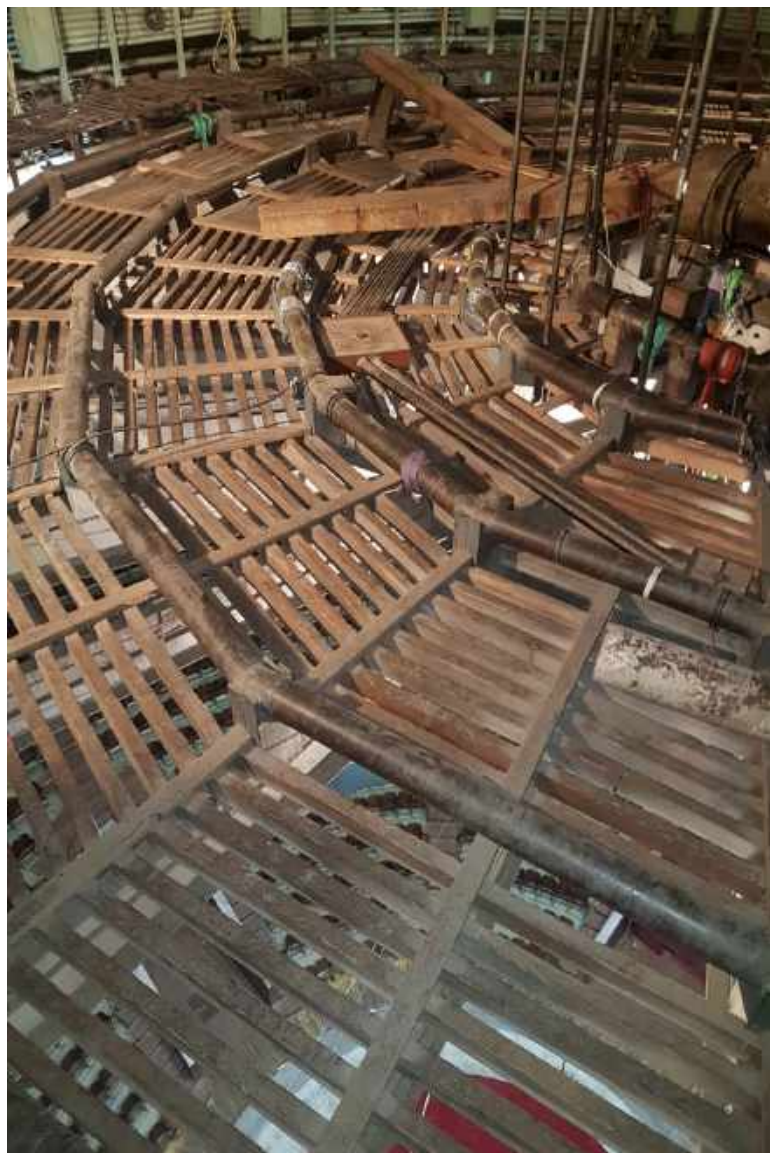
(Picture № 29). Rigging points for circus apparatuses
